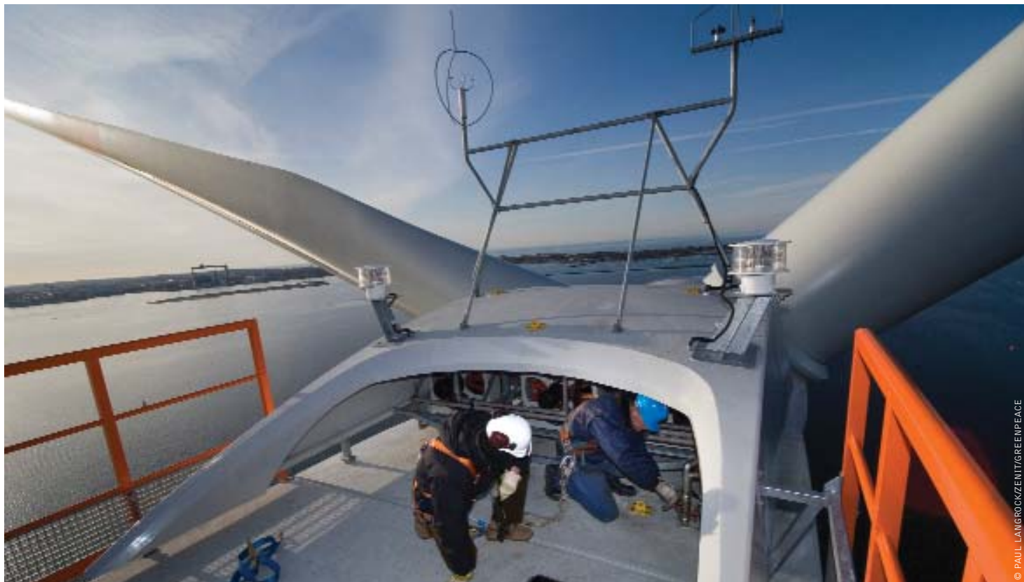
image TEST WINDMILL N90 2500, BUILT BY THE GERMAN COMPANY NORDEX, IN THE HARBOUR OF ROSTOCK. THIS WINDMILL PRODUCES 2,5 MEGA WATT AND IS TESTED UNDER OFFSHORE CONDITIONS. AT LEAST 10 FACILITIES OF THIS TYPE WILL BE ERECTED 20 KM OFF THE ISLAND DARSS IN THE BALTIC SEA BY 2007. TWO TECHNICIANS WORKING INSIDE THE TURBINE.
