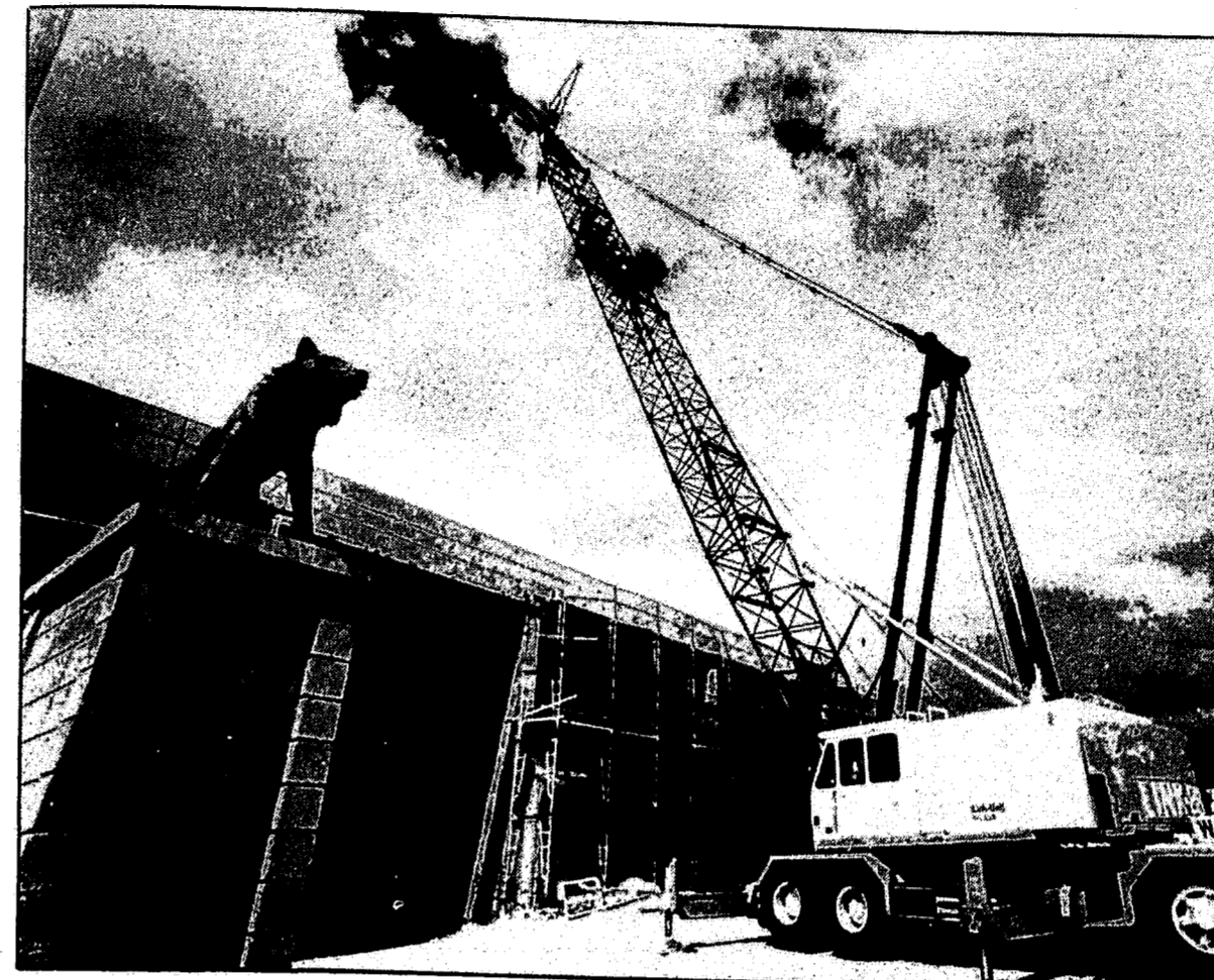
A crane stands in front of Johnson Gym Wednesday helping the construction work that has gone on since the gym renovation began last April. Phase I of the project, which includes new basketball and handball courts, is expected to be completed next March. Phase II, which includes the creation of a new floor and extensive classroom space for the gym is expected to get under way next year if the Legislature approves the funding.
