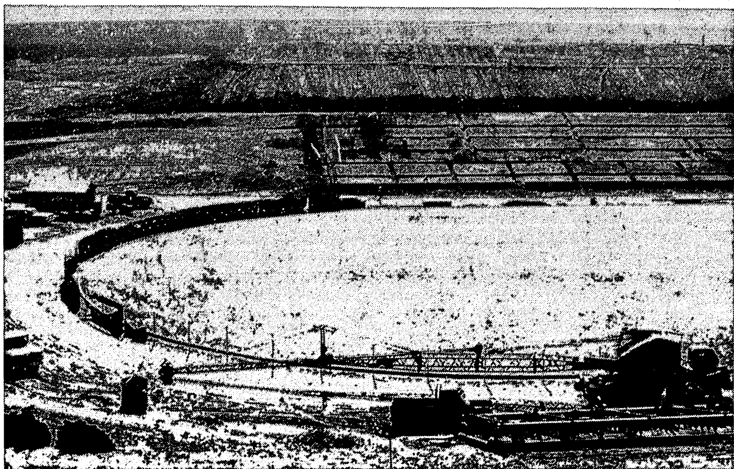
STADIUM CONSTRUCTION entered Phase II last week as officials reported work on the 30,000 seat structure was "on schedule." The Lobos are expected to play their first game in the stadium Sept. 17 with the University of Mexico. See Page 2 for story. (Staff Photo)
