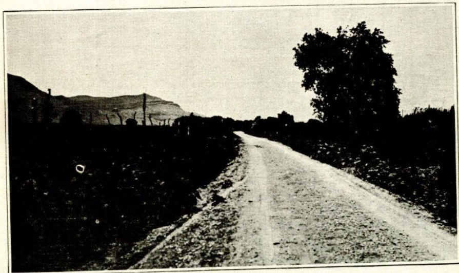
ROAD NEAR HILL STATION, DONA ANA COUNTY (Part of Camino Real—Built by County)
