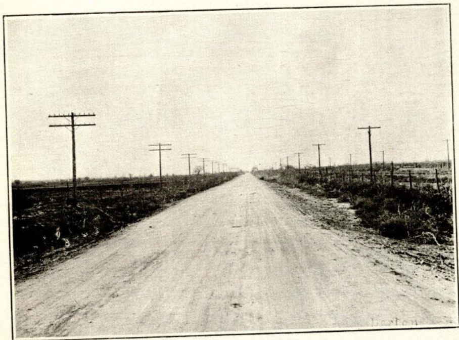
ROAD BETWEEN LAS CRUCES AND MESILLA PARK (State Road No. 1—Built by Dona Ana County)
