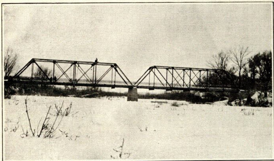
BRIDGE OVER MORA RIVER, NEAR WATROUS (State Road No. 1—Two 120-foot spans—Built by Highway Commission)
