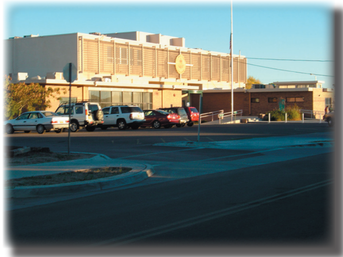
existing courthouse entrance
