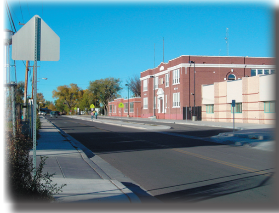
existing view north to Main Street
