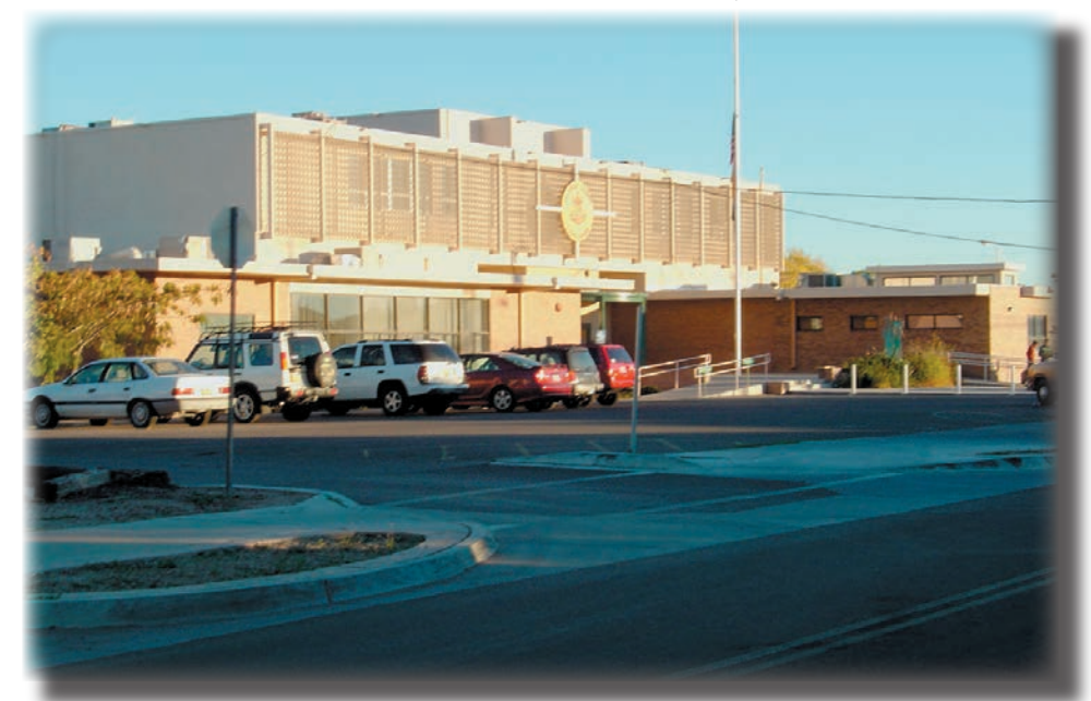
Valencia County Courthouse, 2004
