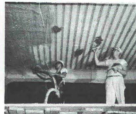
1 Application of Zonolite Direct-to-Steel Fireproofing by machine. Spot troweling only is required.
