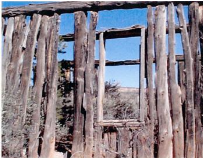
Figure 20: Ruins of a jacal . This was the former home of Luis Trujillo and family near the Arroyo del Oso, in the Cañón del Río de Chama (Photo courtesy of Chris Chavez).
