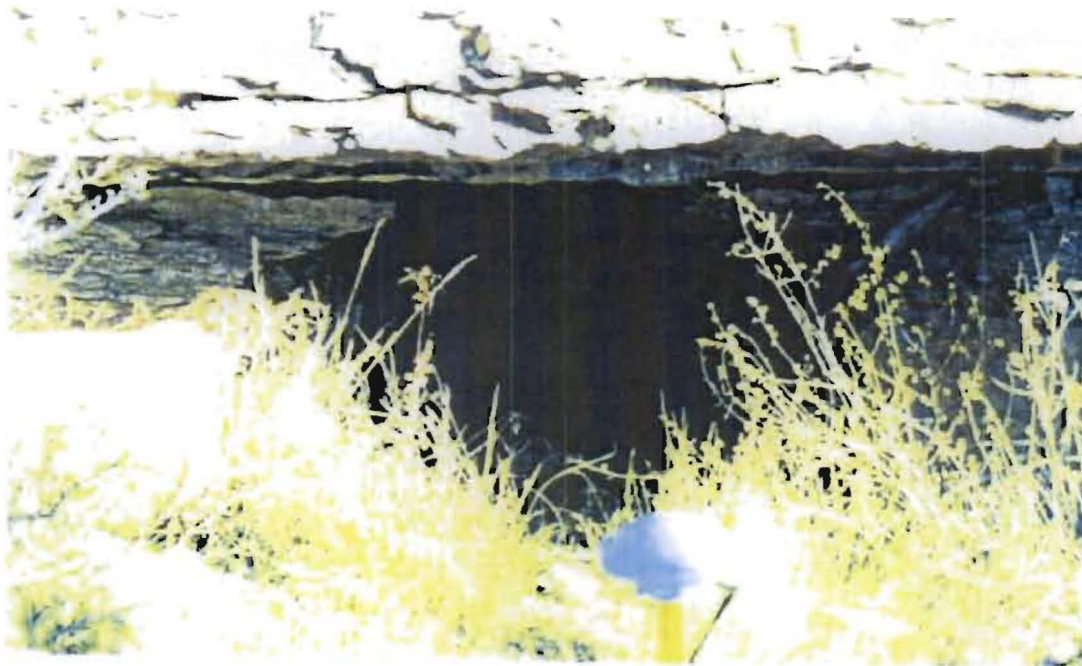
Figure 10a Site 28-9. Horizontal adit. View to the east. GPS instrument antennae in foreground.
