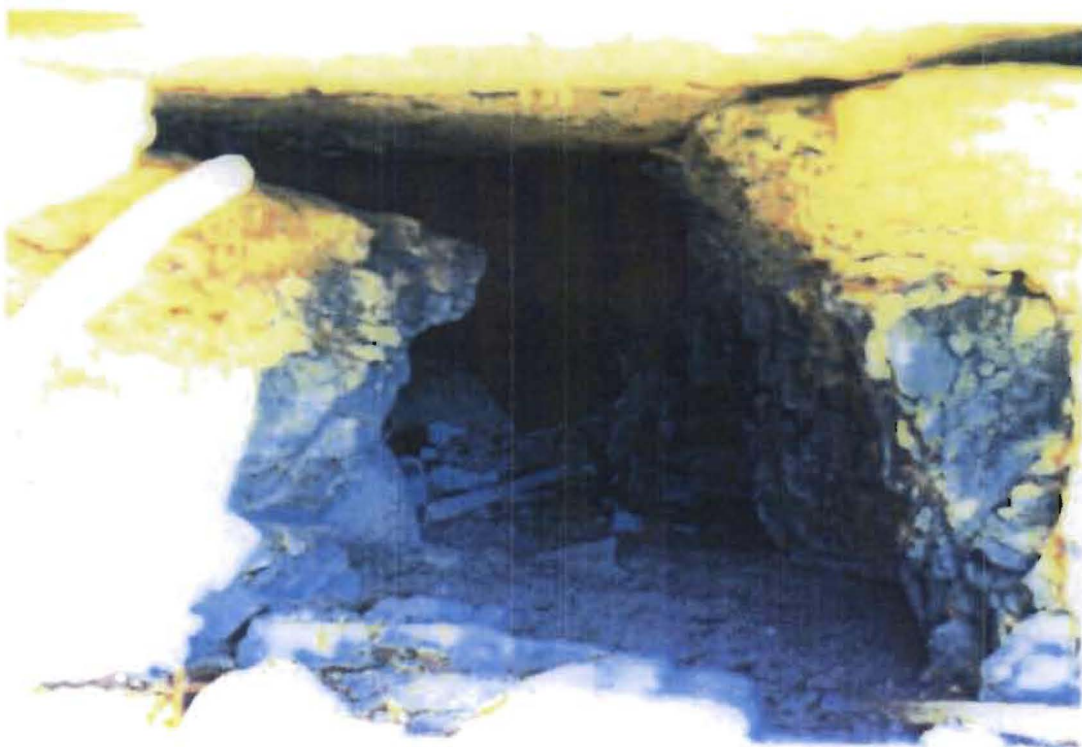
Figure 10b Site 28-9. Closeup of inside of adit. Approximately 5 ft. from ceiling to floor.
