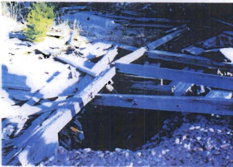
Figure 5b Site 28-4. Closeup of the top of the main shaft.
