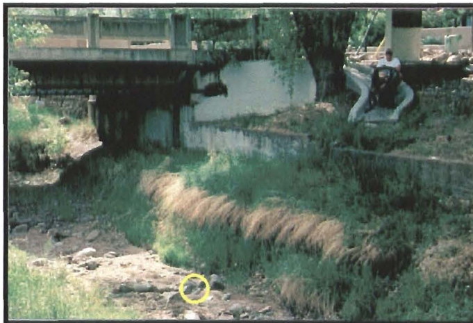
Photograph 2 – Location B – Below Delgado St. and Arroyo Saiz
