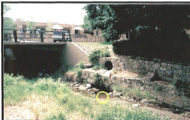
Photograph 3 – Monitoring Location C – Below Santa Fe Trail
