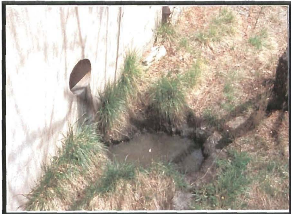
Photograph 2 Typical drainage outlet in the urban reach of the Santa Fe River
