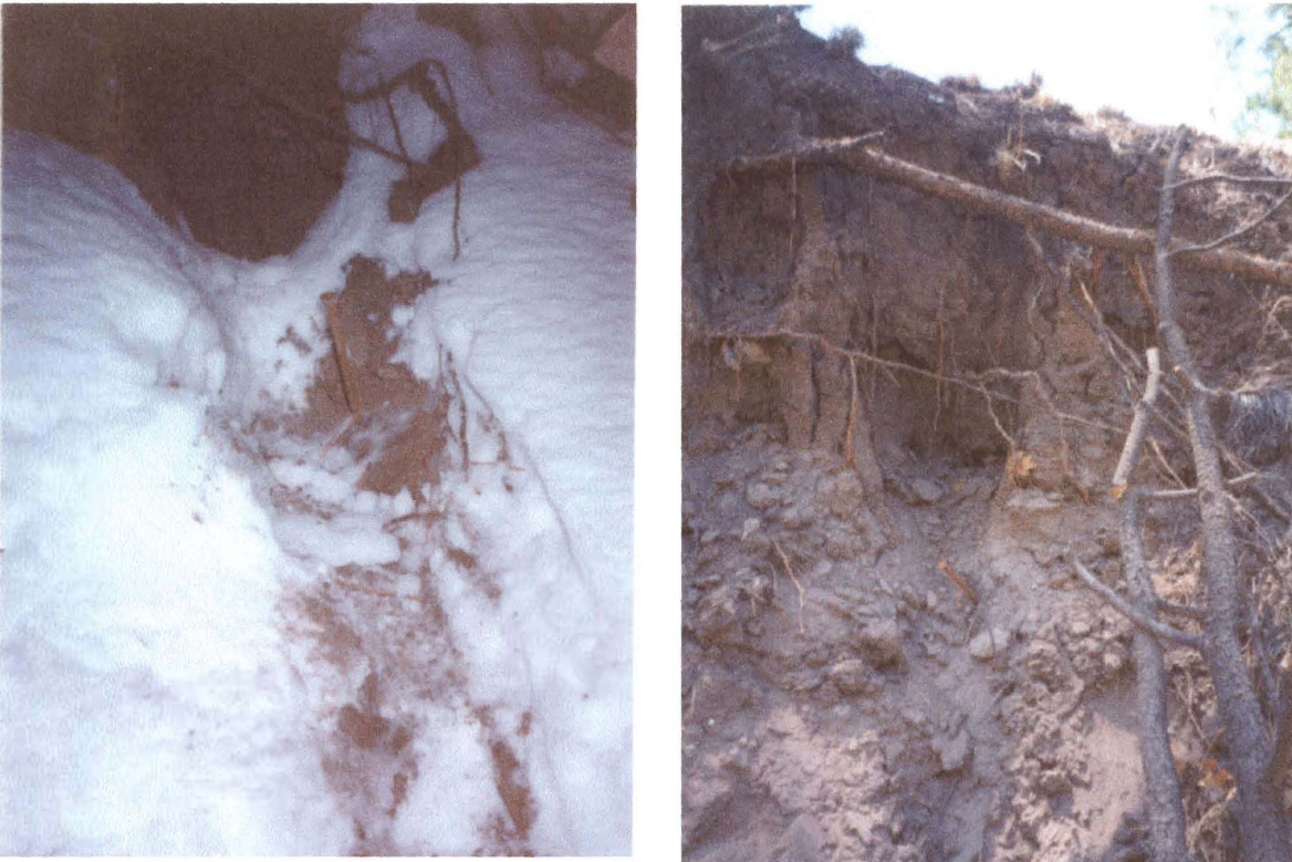
Figure 4- 7 Site 3A - erosion pin 2 The picture on the left was taken in January. The picture on the right was in March; notice the sediment on top of the washer.
