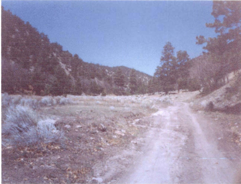
Figure 5-2 When the stream channel flows, water often floods Forest Road 59A in several different locations throughout the canyon.
