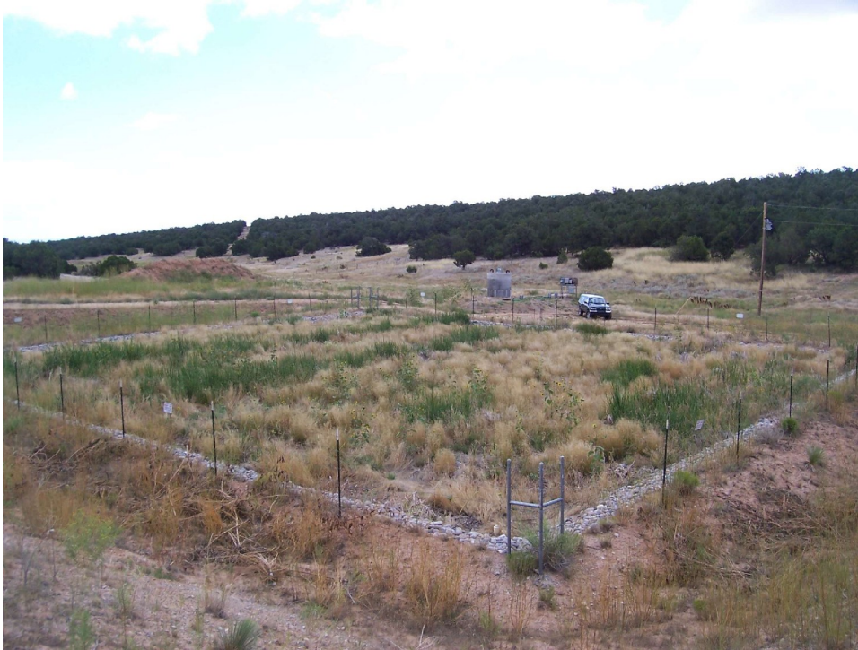
Figure 15. Prairie Hills Constructed Wetland - August 2007
