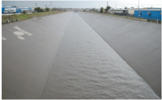
Figure 6: The North Diversion channel after a rain event.
