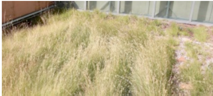
Figure 22: A “living roof” at the School of Architecture and Planning, University of New Mexico. The term “living roof” is used instead to more accurately reflect the native plant pallet used. This roof was designed to be irrigated with either potable or harvested water, and is currently being monitored to quantify benefits and hydrologic activity.
