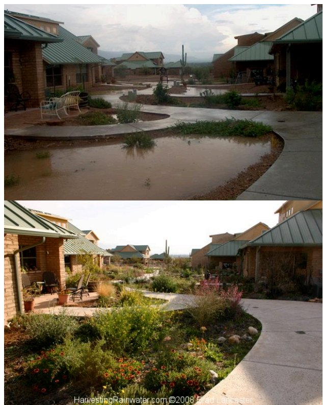
Figure 20: Rain gardens at the Milagro Co-housing development outside of Tuscon, AZ. Top photos is before native vegetation was planted. Photo source: Brad Lancaster, www.harvestingrainwater.com
