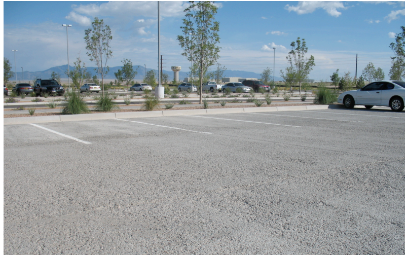
Figure 21: Porous pavement. Mesa del Sol, Albuquerque, NM.
