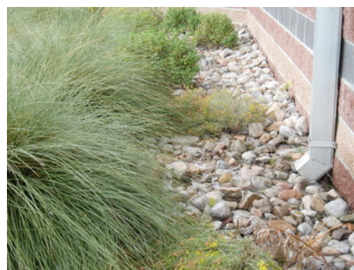
Figure 19: An infiltration planter. Downspout drains to vegetation area at Pavilions Shopping Plaza, Albuquerque, NM.
