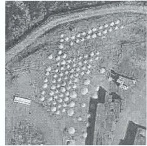
(Concrete Capped Disposal Shafts)
