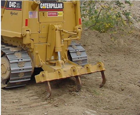
Figure 3. Tines on the back side of a dozer, or similar agricultural tillage equipment, when applied on the contour and perpendicular to water flow, can increase infiltration and reduce erosion. (Erosion Control Network)
