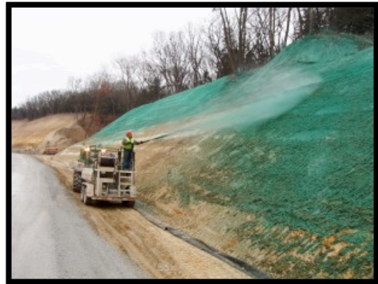
Seed being hydraulically applied to slope
