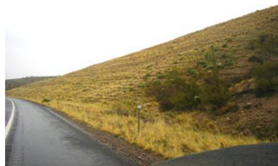
Mini-benching with seeded vegetation
