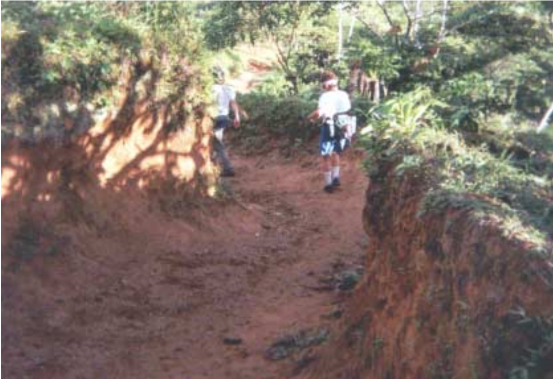
Fig 2. An eroded portion of the road to Miramar.
