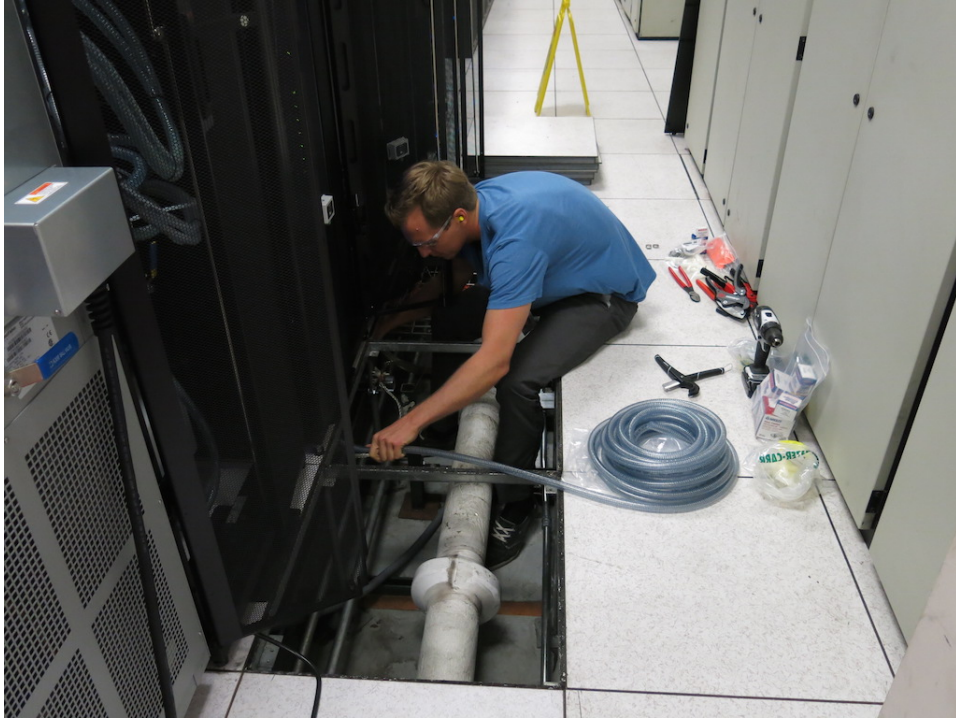
Figure 5: Chris from Chillydyne measuring the tubing for rack to rack connections.
