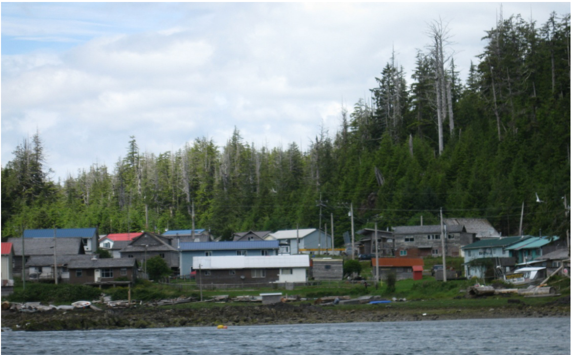
Figure 15. Example of the close quarters and aging condition of homes in this community. Lottis, 2010.
