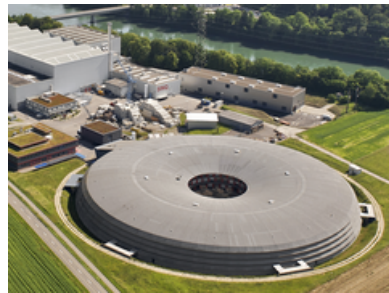
Figure A.10: The Swiss Light Source (SLS) at the Paul Scherrer Institut is a third-generation synchrotron light source. With an energy of 2.4GeV, it provides photon beams of high brightness for research in materials science, biology and chemistry. .
