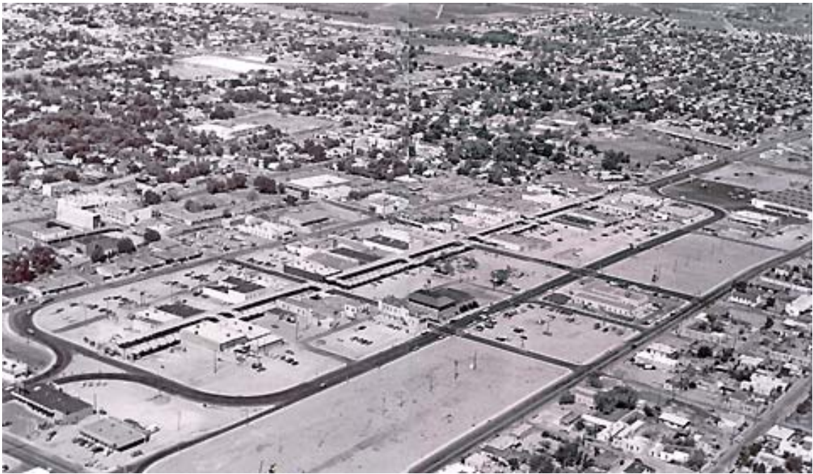
Ill. 6-3. Aerial View of Downtown Las Cruces after Urban Renewal ( Illustration courtesy Las Cruces Blog: News, Photos, History, http://lascrucesblog.com/category/history/page/2/ )
