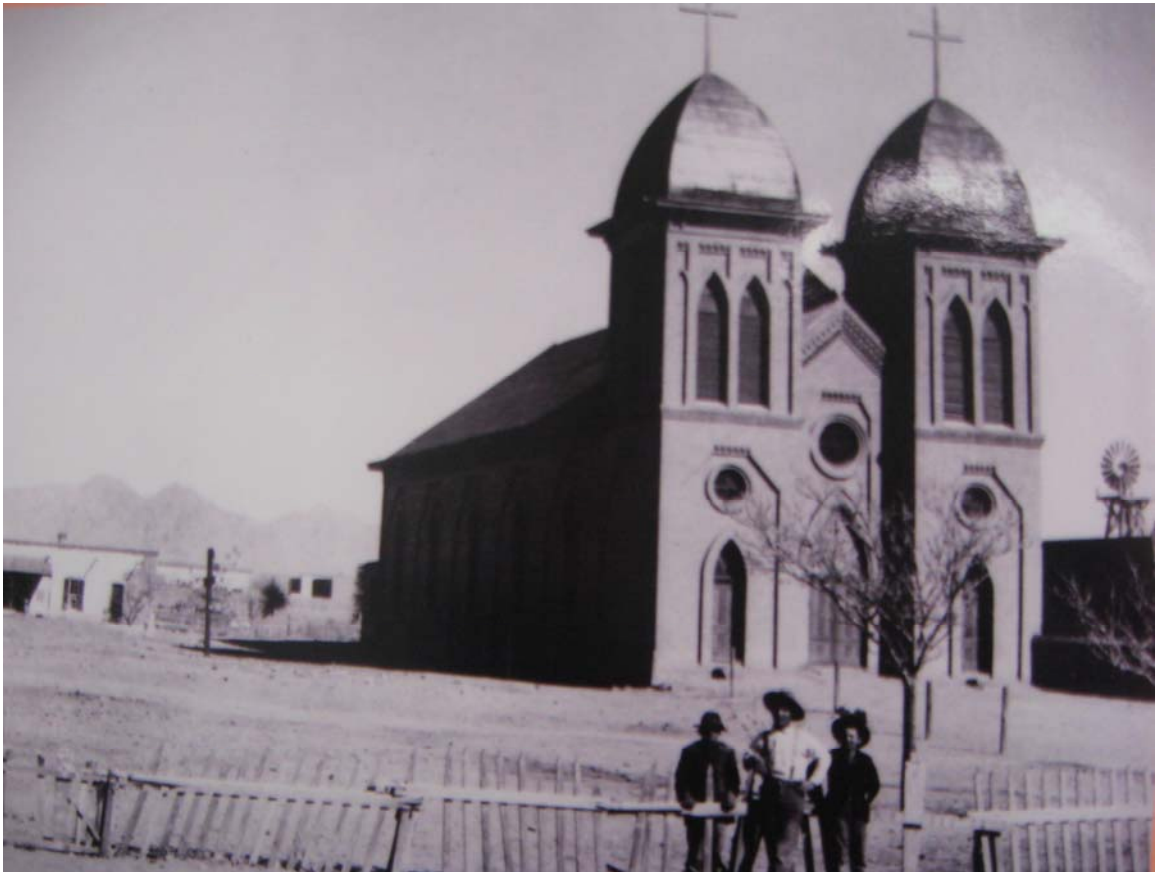
Ill. 2-1. St. Genevieve Church Prior to the Addition of Buttresses to Exterior Walls, date unknown
