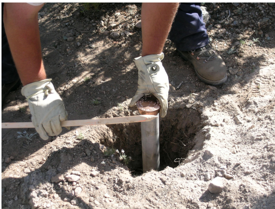
Figure 35. Setting the newly-surveyed corner brass cap.
