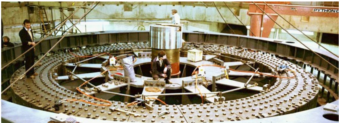
Figure 1.10: 1 MWh storage capacity flywheel in Culham, UK [13].
