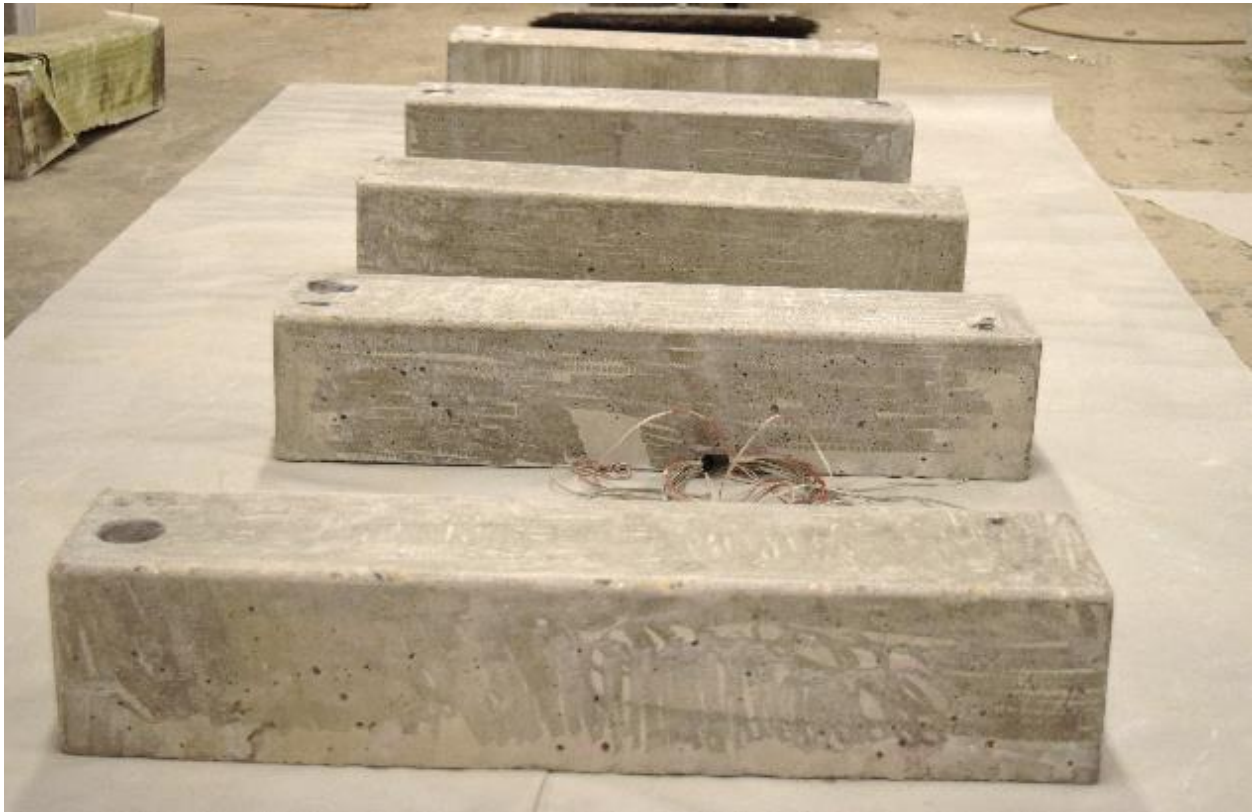
Figure 3.10: Grinded RC beams ready for FRP wrapping
