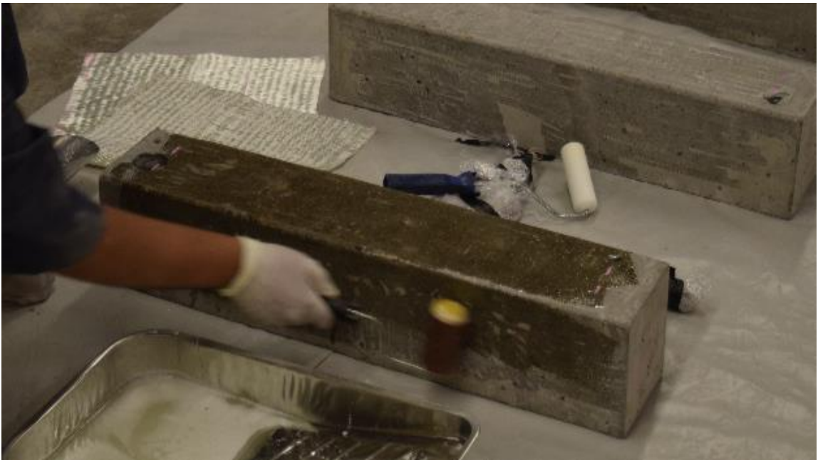
Figure 3.13: Prime coat with adhesive before GFRP wet-layup
