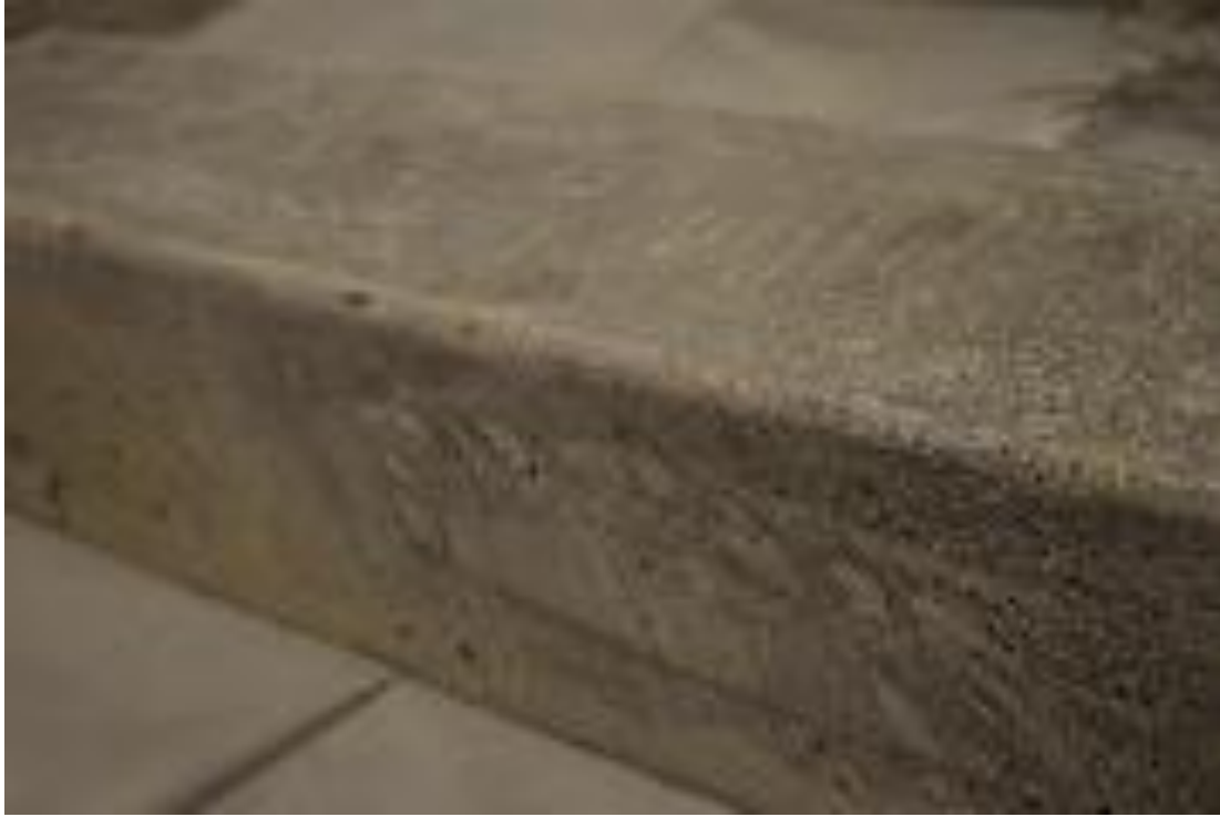
Figure 3.11: RC Beam showing rounded edge prior to GFRP wet-layup application
