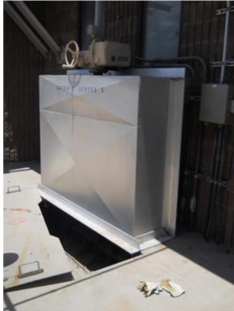
Figure 26 Gate Cover and Plate Over Effluent Channel
