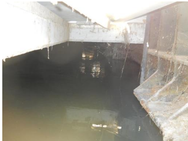
Figure 28 PTF Channel Looking Downstream - Slide Gate on Right
