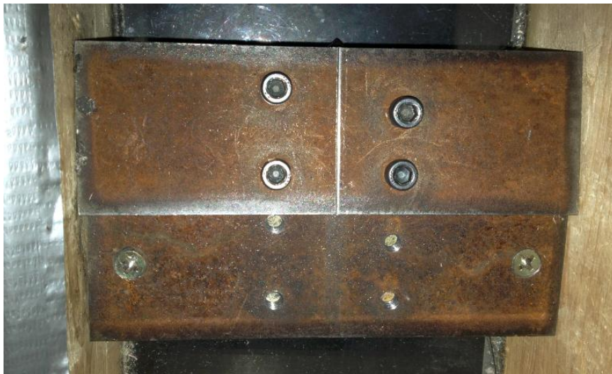
Figure 3.2.3 Details of the clamp
