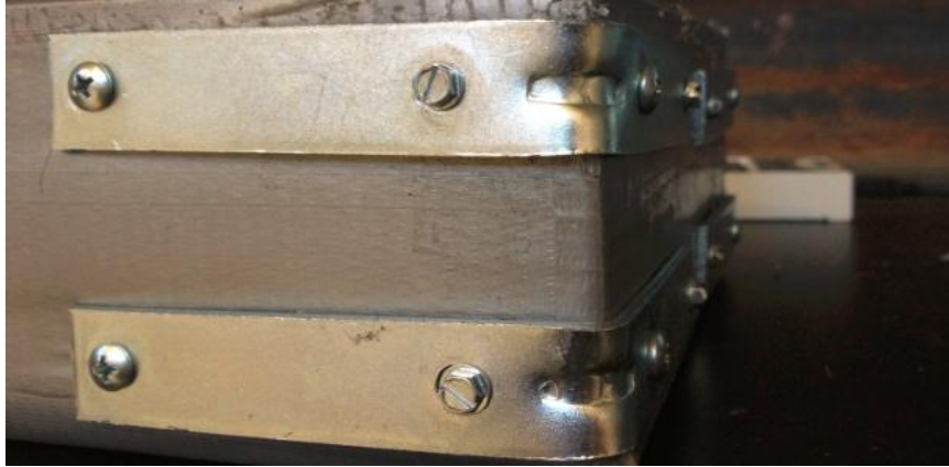
Figure 3.4.5.2 Details of the stiffened frame corners
