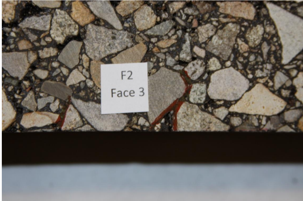
Figure 6.6 Fatigue Crack Propagating Upwards in HMA Beam Sample SP-III-F2
