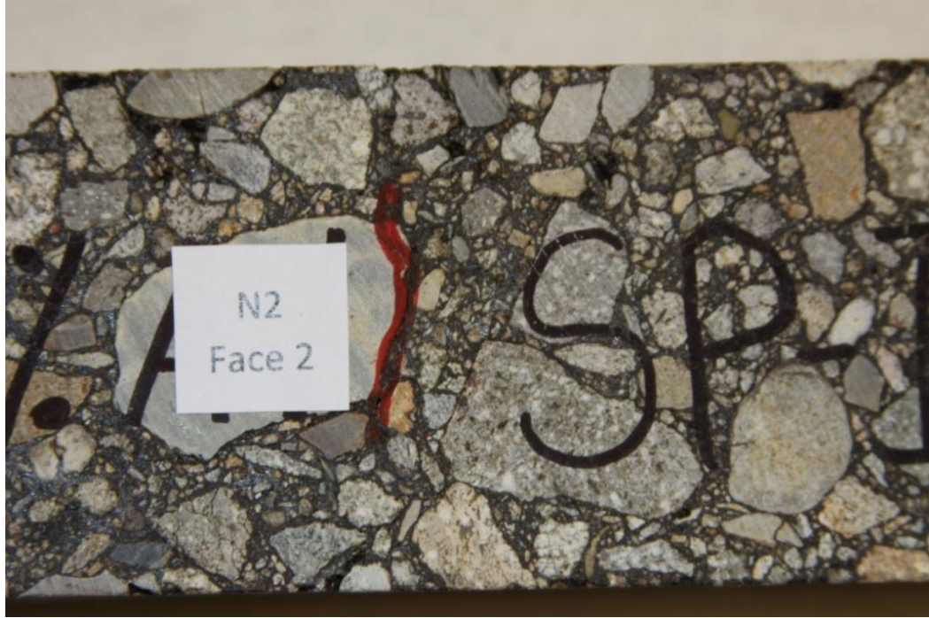
Figure 6.4 Fatigue Cracking in HMA Beam Sample SP-II-N2
