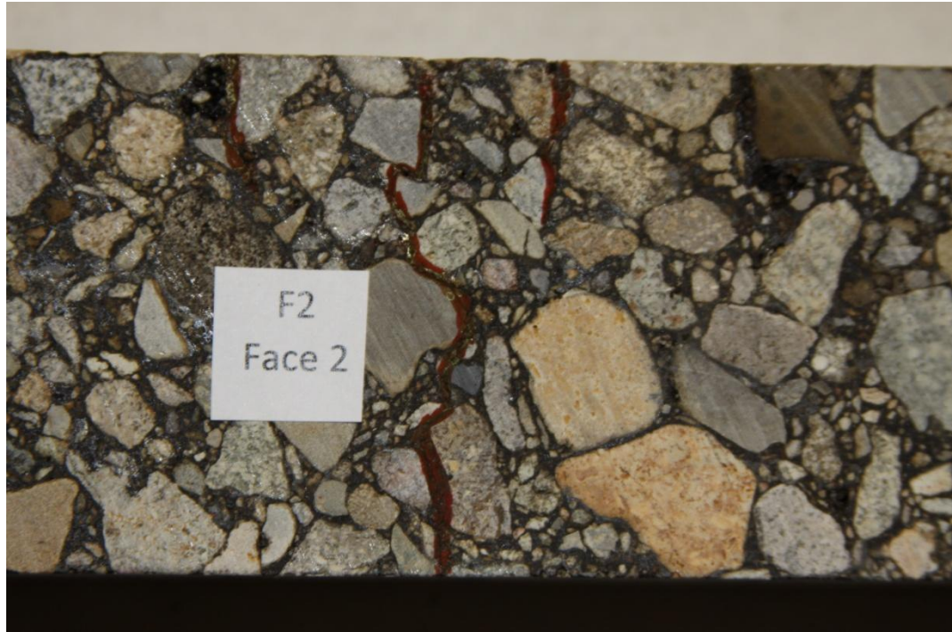
Figure 6.5 Fatigue Cracking in HMA Beam Sample SP-III-F2
