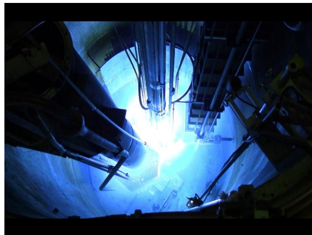
Figure 1 – Three Experimental Cavities at the Annular Core Research Reactor Facility (ACRRF) During a Pulse
