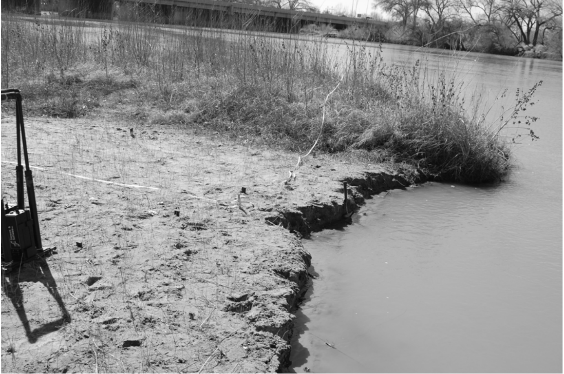
Figure 10 - Northern most edge of the GPR survey site, directly along the Rio Grande. Survey markers, string, the non-conductive tape measure and GPR equipment are visible on the left side of the photograph. Hand probing into the study site after data collection confirmed that depth to water was only several centimeters throughout the study site.
