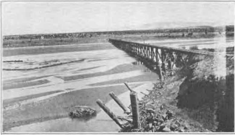
Figure 18. Aqueduct over the Jemez river. This permits water taken from the Jemez, above the Salado, to be used on Zia Indian land, south of the Jemez.
