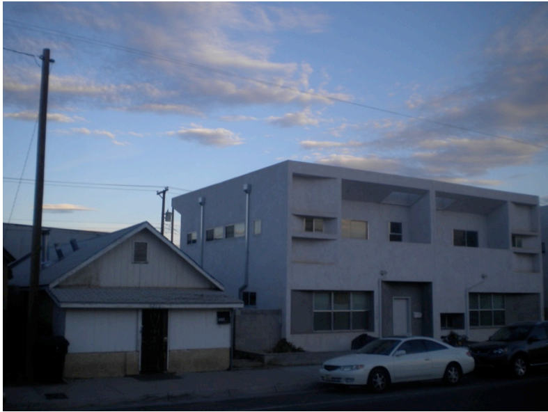
Newer condominiums dwarf an older row-style house on 3 rd Street in Barelaz.
