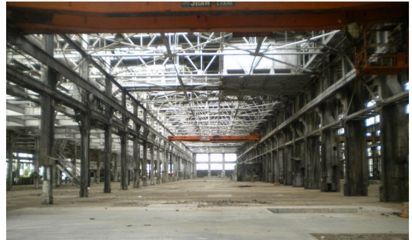
The inside of Albuquerque's Rail Yard Machine Shop are 160,000 square feet in size.
