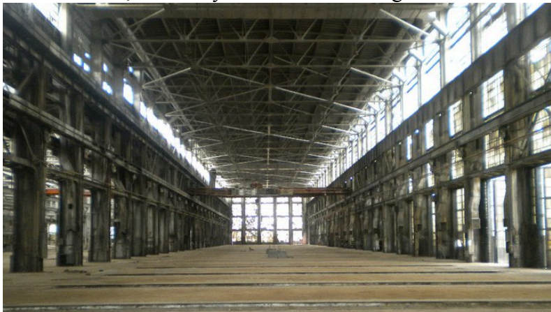
Interior of the Rail Yard Machine Shop
