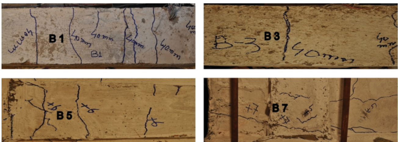
Figure 17. Crack patterns in beams attributable to pre-loading (+3, +4, +6 and +7 markings on the beams indicate cracks initiated at displacements of 30 mm, 40 mm, 60 mm and 70 mm, respectively)
