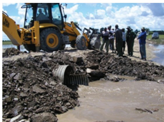
Installation of a temporary culvert during flood
