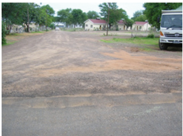
Intersection of paved and gravel roads
