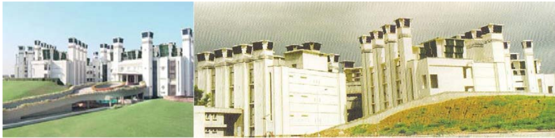
Figure 2.19. Passive down draught cooling in Ahmedabad. 17
