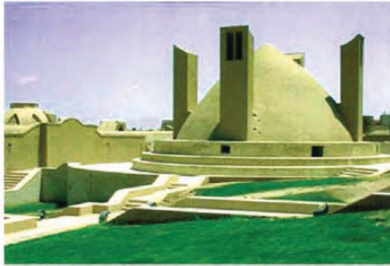
Figure 3. 19. Ab anbar or “water reservoir”. 32
