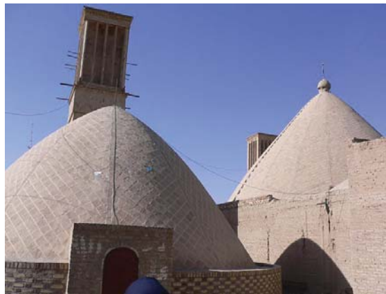
Figure 3.18. Qanats used in conjunction with a wind-tower can provide cooling as well as a water supply. Wind-towers of Ab-Anbar (An Ab-Anbar is a traditional Qanat fed reservoir for drinking water in Persian antiquity.) 31
