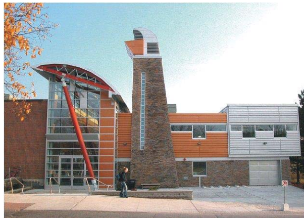
Figure 3.9. Wind catcher at Sir Sanfred Fleming College, Peterborough, Canada. (Source: Loghman Azar, Line Architects, Toronto)
