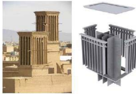
Figure 3.13. An example of wind-catcher and internal blades wind-catchers in Iran. (A'zami, 2005)
