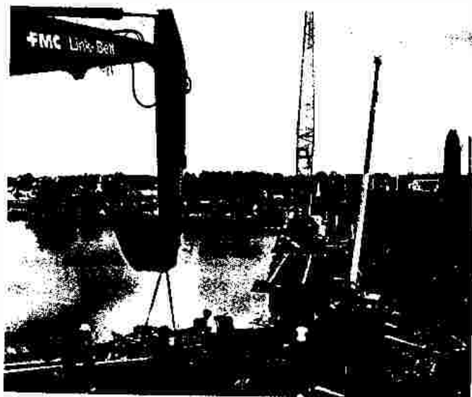
Route 46 bridge construction
