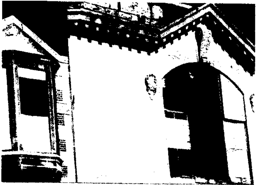
The view is right through the roof of the crumbling Casino
