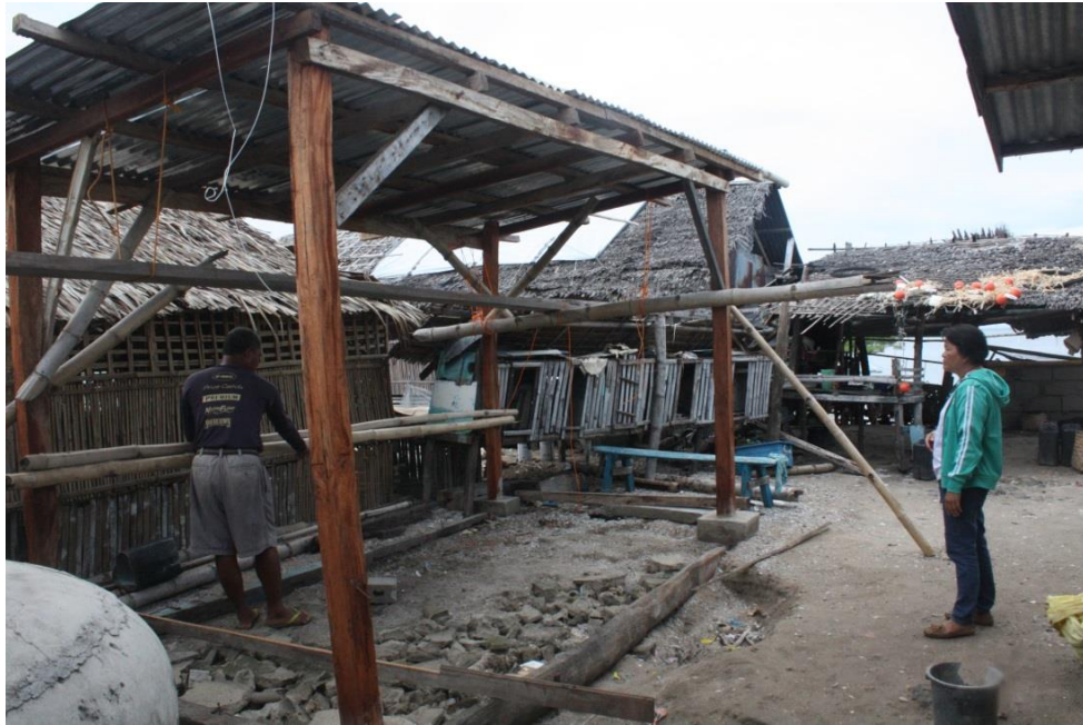
Figure 3.3 Construction of drying shed. Photo by: D. Fenlon.
