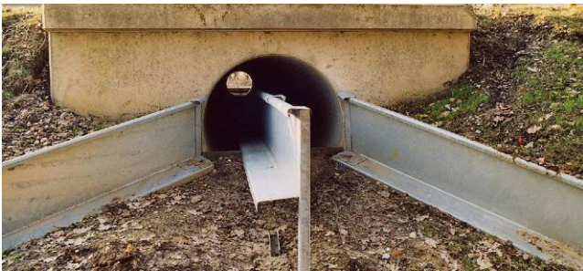
Figure 39. Tunnel under road to permit safe passage of the European Common Toad Bufo bufo to and from its breeding grounds. Photo by Christian Fischer, through Wikimedia Commons.
