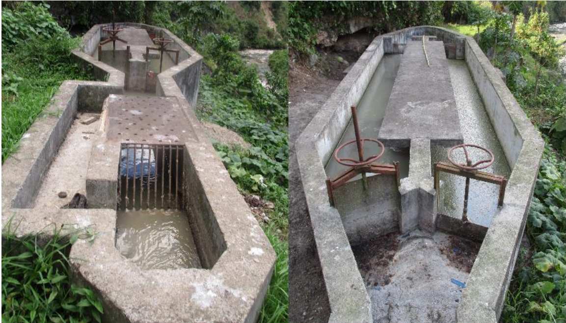
Figure 1.4: Preliminary treatment unit in Leymebamba WWTP. Left image shows whole unit with bar screen in foreground. Right image shows grit chamber. Photos by author.
