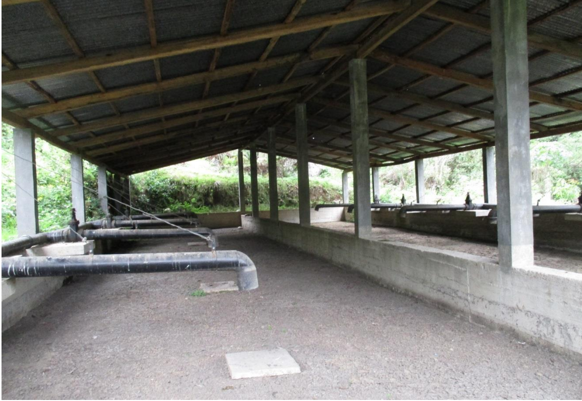
Figure 1.7: Sludge drying beds in Leymebamba. Photo by author.
