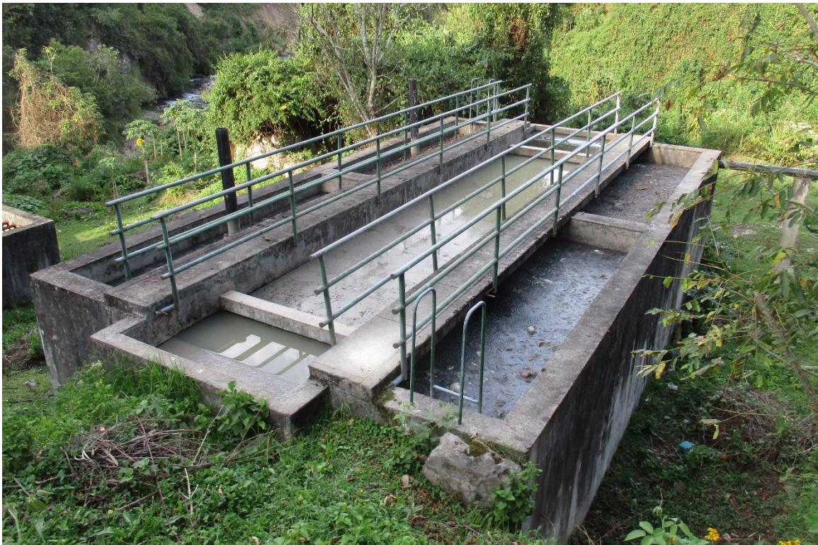
Figure 1.5: Imhoff tank in Leymebamba. The middle chamber is the sedimentation chamber, the sides are scum chambers, and the bottom which is not visible is the digestion chamber. Photo by author.
