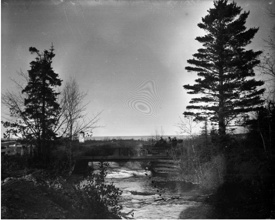
Figure 20. Bridge towards the end of period of use. Note log crib abutment and Model T driving across. Unknown date. Image courtesy of the Michigan Historical Center, Michigan Iron Industry Museum.
