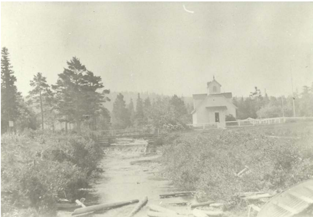
Figure 9. Photograph showing dormers added and redesigned fencing. Note log crib bridge abutments. 1910. Image courtesy of the Michigan Historical Center, Michigan Iron Industry Museum.
