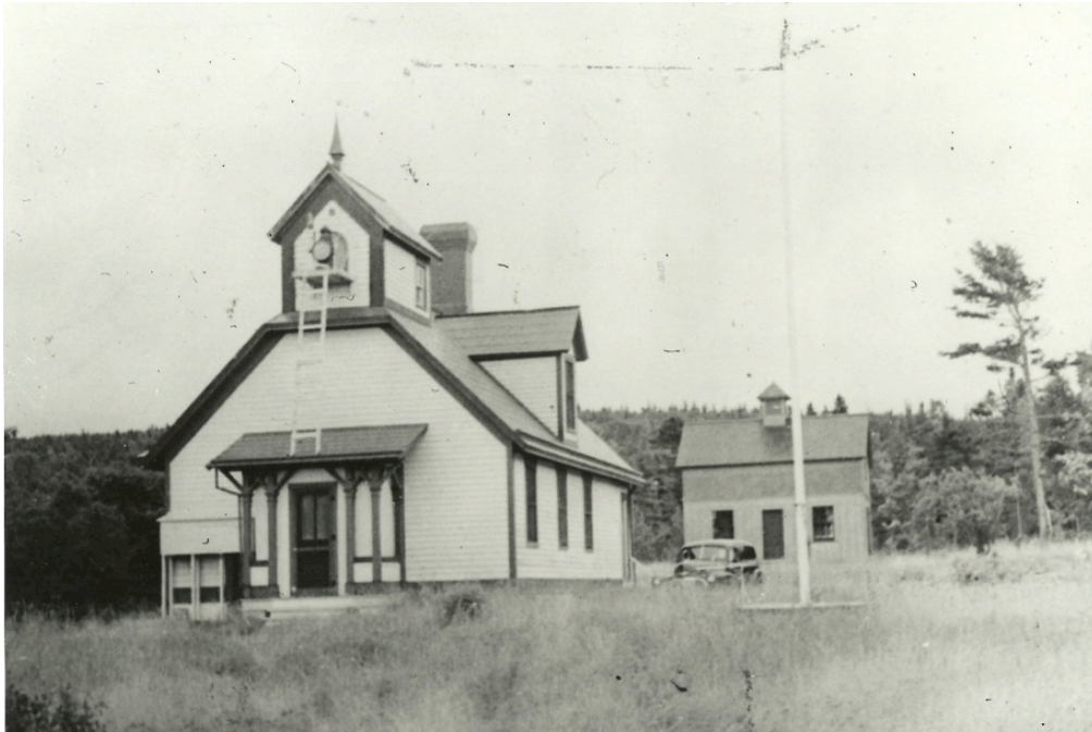
Figure 10. 1945 Photograph showing electric lamp mounted outside of original light bay. Also note lack of fencing. Image courtesy of the Michigan Historical Center, Michigan Iron Industry Museum.
