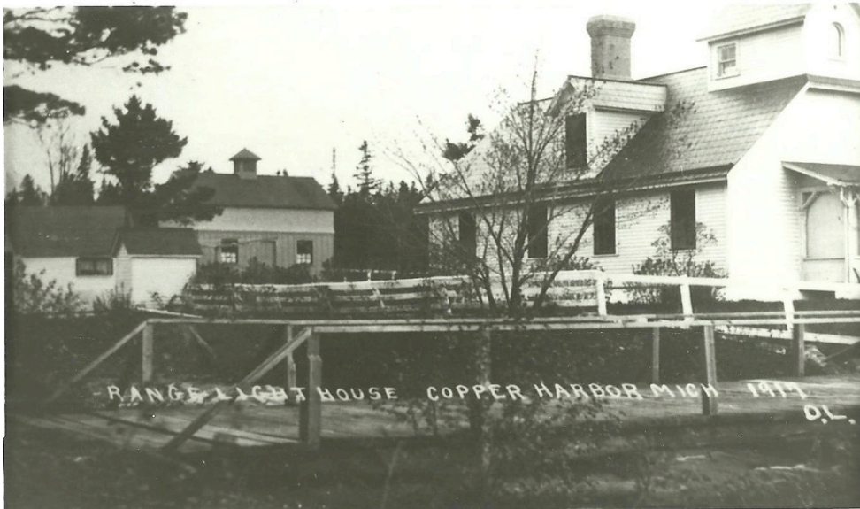
Figure 12. Earliest photograph showing the barn. Also note privy and washhouse to left with white siding. Bridge still in use, appears to have split log decking. 1917. Image courtesy of the Michigan Historical Center, Michigan Iron Industry Museum.
