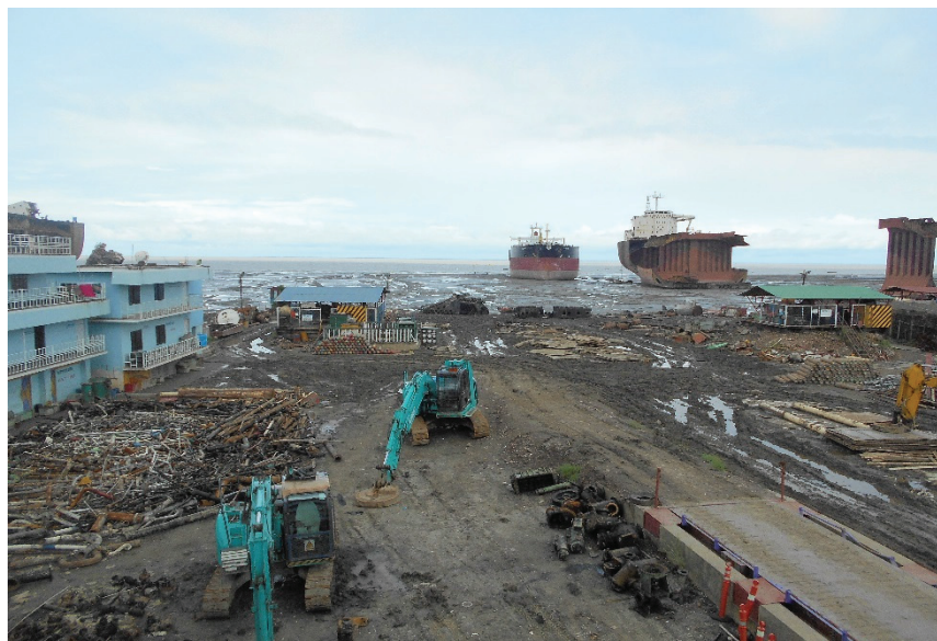
Figure 3.1. Shipbreaking yard, Chittagong, Bangladesh
