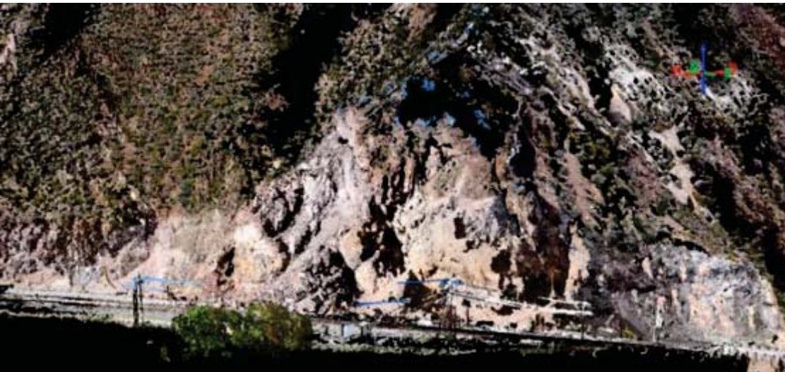
FIGURE 4-6: TERRESTRIAL LIDAR POINT CLOUD OF STUDY SITE SLIDE 1. THE RAILROAD CAN BE SEEN AT THE TOE OF THE SLOPE. THERE IS A HOLE IN THE IMAGE INDICATED WHERE THE LIDAR SCANNER COULD NOT SEE, BECAUSE OF A CHANGE IN THE ANGLE OF THE SLOPE.
