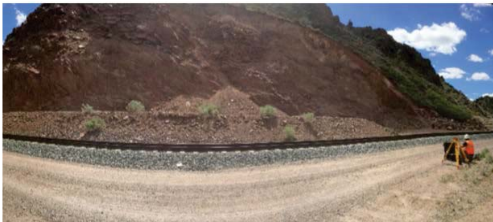
FIGURE 2-6: TERRESTRIAL LIDAR SCANNER USED AT THE STUDY LOCATION IN SOUTHERN NEVADA. THIS IS A STATIC SCANNER, AND WAS SET UP TO SCAN THE ENTIRE SLOPE HEIGHT. LOCATION MUST BE ADJUSTED TO SCAN THE ENTIRE LENGTH OF THE
