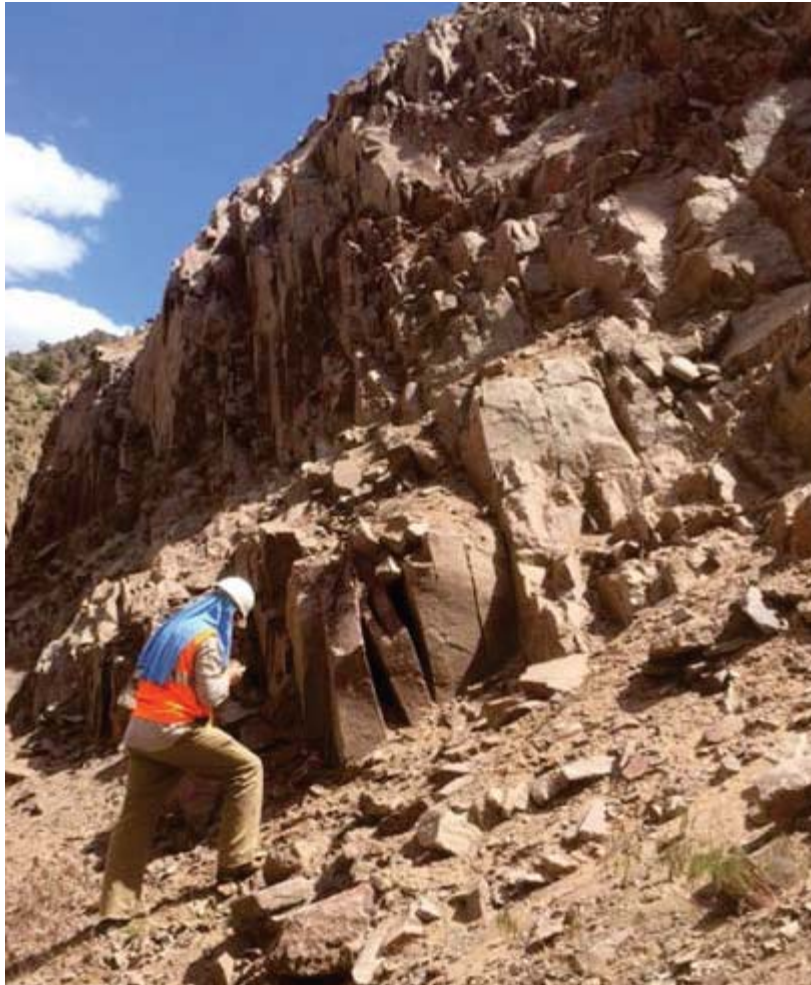
FIGURE 3-7: ROCK STRUCTURES AT SLIDE 2 CAN BE SEEN IN THIS PHOTOGRAPH. ONE OF THE MAJOR STRUCTURES IN THE ALMOST VERTICAL PLANE. ROCK BLOCKS APPEAR TO MOSTLY BE FAILING ALONG THIS PLANE.
