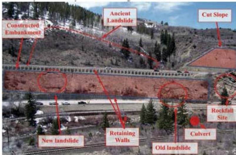
FIGURE 2-1: SCHEMATIC OF GEOTECHNICAL ASSETS AS DEFINED BY THE FEDERAL HIGHWAY ADMINISTRATION (10). THERE ARE MANY GEOTECHNICAL ASSETS PRESENT ALONG TRANSPORTATION AREAS. THIS DIAGRAM SHOWS THE INFRASTRUCTURE ASSETS ARE INSEPARABLE FROM THE GEOTECHNICAL ASSETS THEY ARE BUILT UPON.
