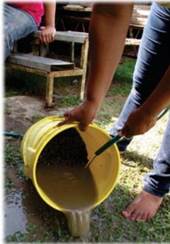
K. Instructions and photo to aid in the washing of sand.
