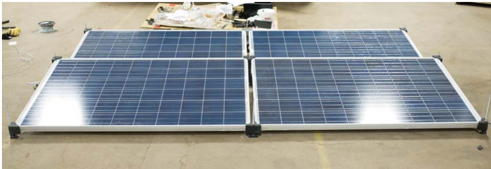
Figure 4.6: Assembly of 1kW X-wire racking system.
