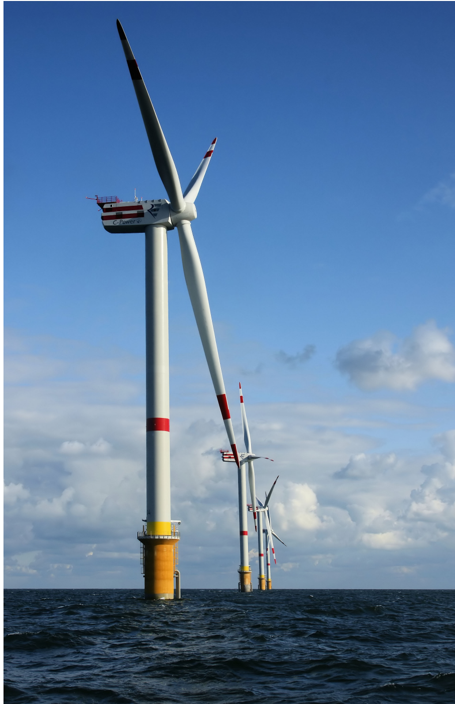
Figure 1.2. The REpower M5 5-megawatt turbine, with a rotor diameter of approximately 126 meters, [taken from Wikimedia Commons 20].
