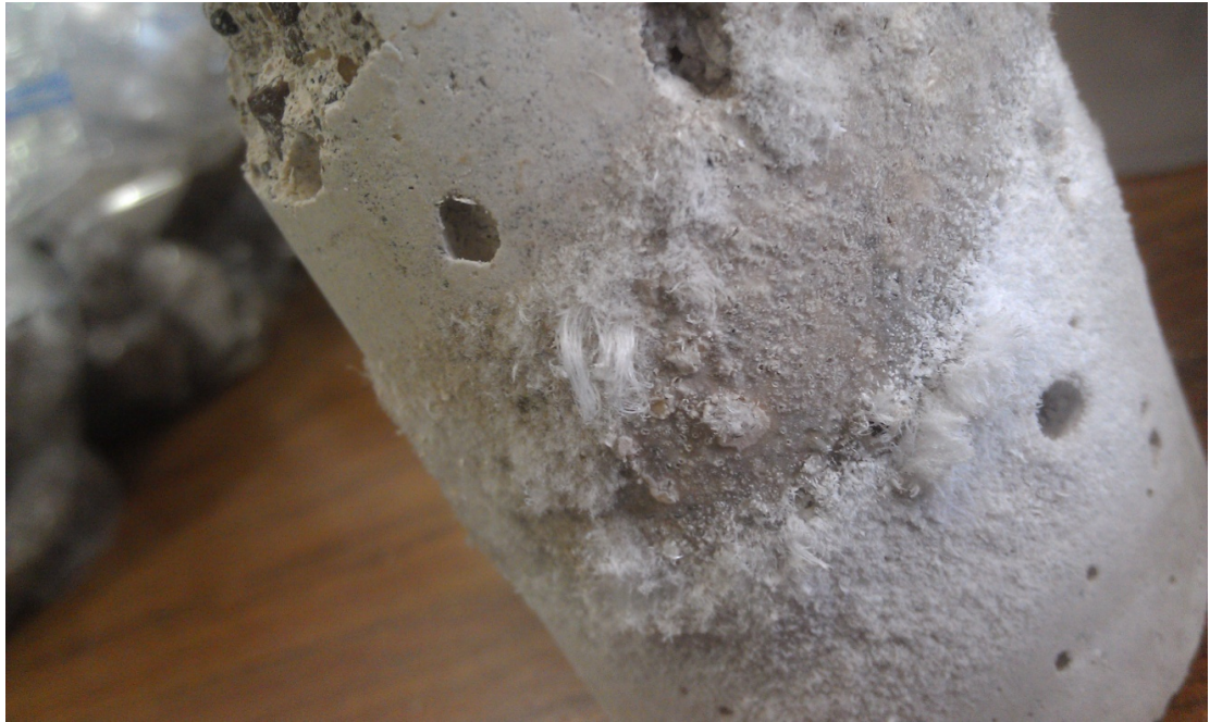
Figure 4.19. White growth on the surface of the C.5.80 mortar during storage.
