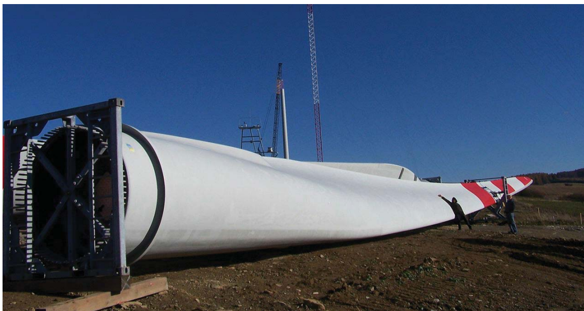
Figure 1.4. REPower 5M wind turbine blades. Wind farm installation at Bukowsko-Nowotaniec, Poland. Picture taken by Korona B. Copyright statement in Appendix A.
