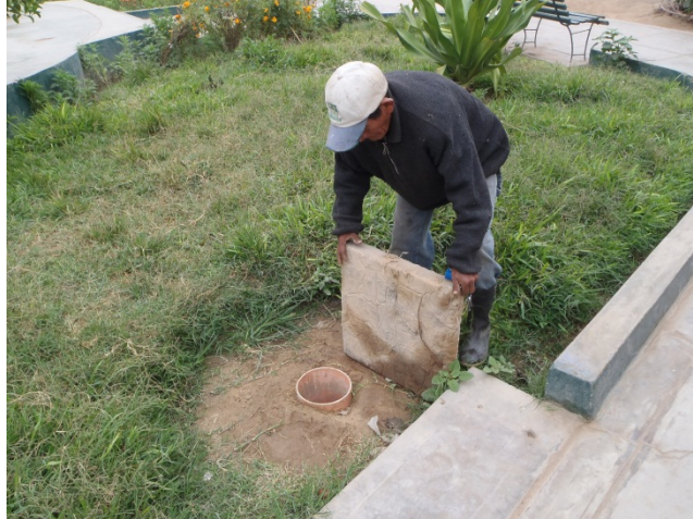
Figure 9 The Operator must Manually Open Valves for Branches of the Water Network (O'Neill, 2012)
