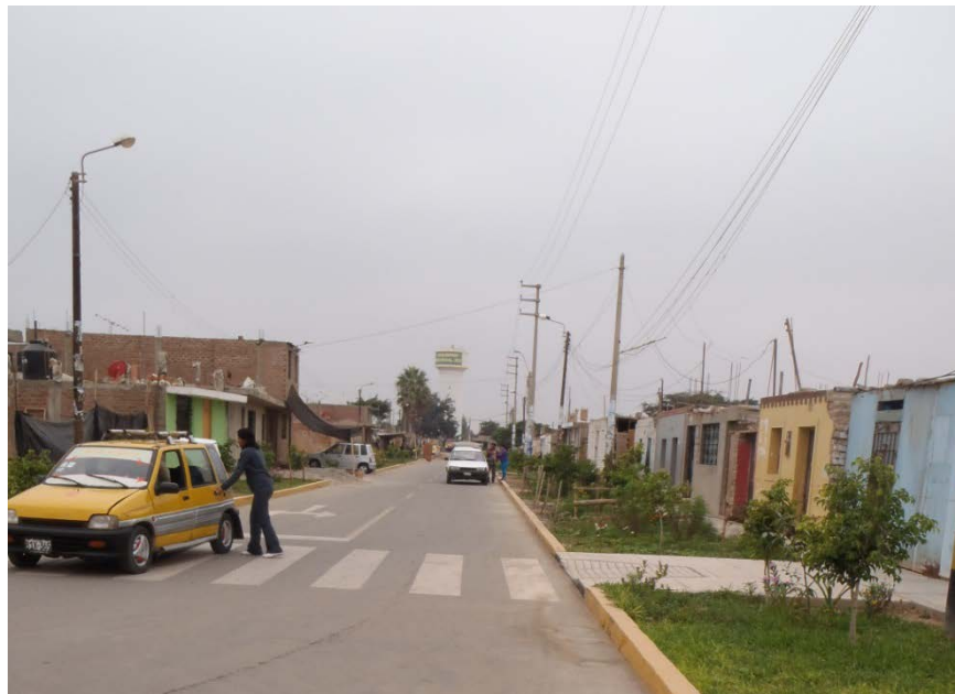
Figure 5 Cerro Prieto, View of Elevated Water Tank (O'Neill, 2012)
