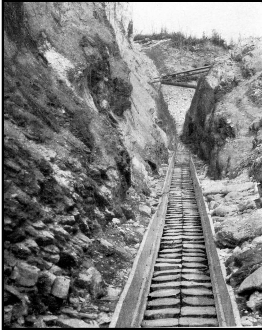
Figure 3.9: Sluice with cobblestone riffles in Alaska (Purinton 1905:Plate XXIV)
