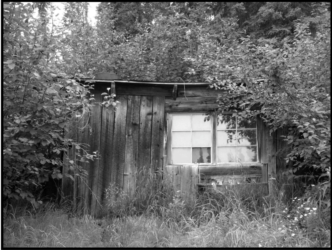
Figure 6.7: Chatham Creek Site Engine House (Baeten: 2011)
