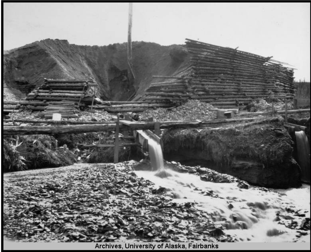
Figure 6.4: Washing a winter dump (Courtesy of University of Alaska Fairbanks, Alaska and Polar Regions Collection, Albert Johnson Collection, Accession #UAF-1989-166-22)
