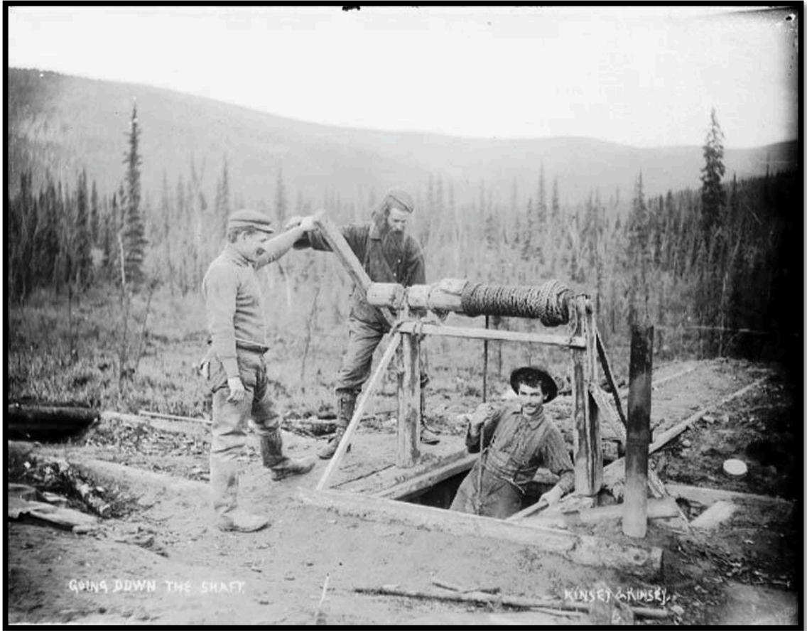
Figure 5.10: Hand windlass above shaft (Courtesy of University of Washington Libraries, Special Collections, William E. Meed Collection, UW16633).
