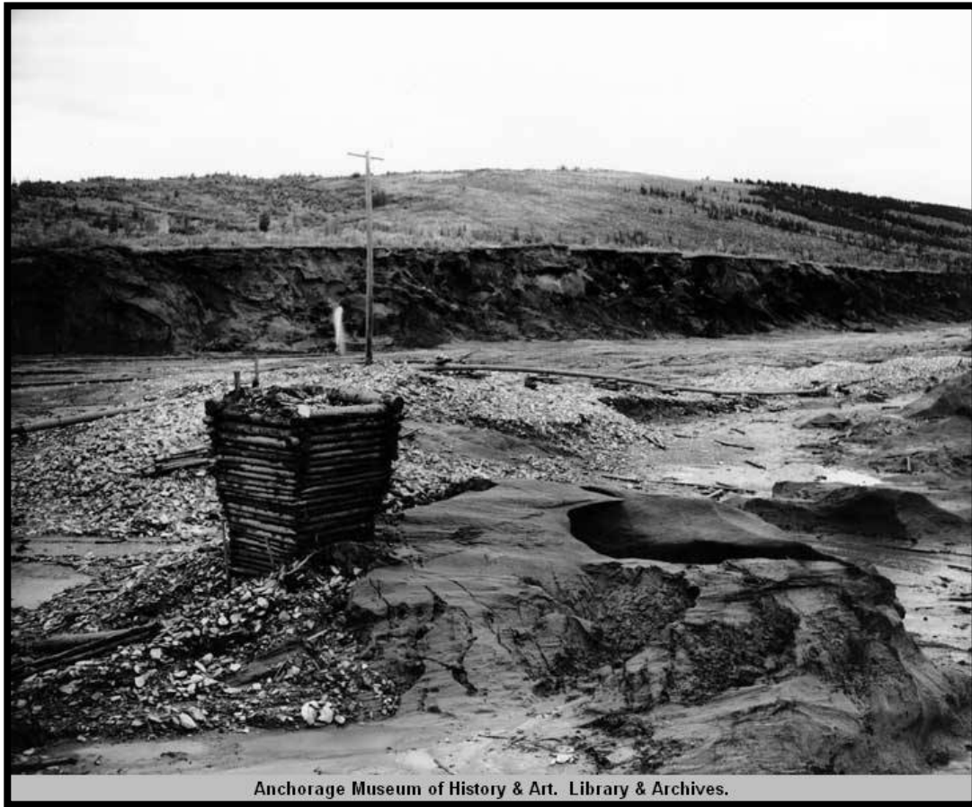
Figure 6.17: Thawed and prepared dredging area, showing intact cribbed shaft from prior drifting (Courtesy Anchorage Museum of History & Art, Ickes Collection, Accession #B75-175-259)
