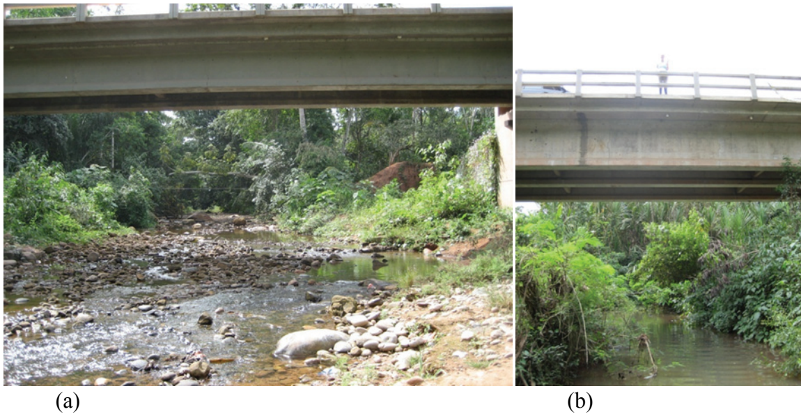
Figure C 4. The monitoring locaitons of (a) the Mapuruchuqui watershed and (b) the IBTA watershed. The roughness values for the Mapuruchqui watershed were determined as n_{\text{floodplain}}=0.0475 (scattered brush) and n_{\text{channel}}=0.04 (cobbles). The roughness values for the IBTA watershed were determined as n_{\text{floodplain}}=0.11 (dense brush) and n_{\text{channel}}=0.039 (clean, irregular). Photographs by author.
