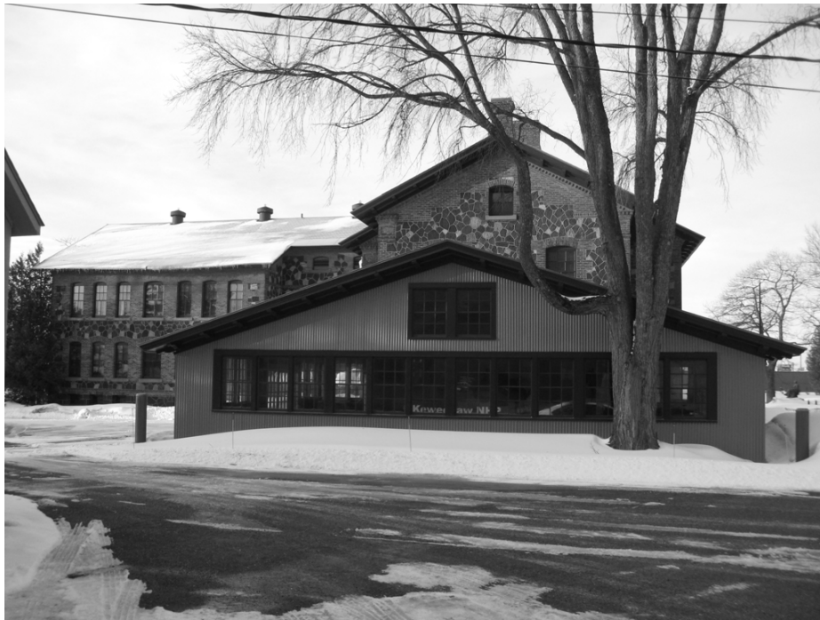
Figure 3.13: View of KNHP headquarters looking south. In the foreground is the north addition payshed, with the east addition also present. Photograph by author, 2011.
