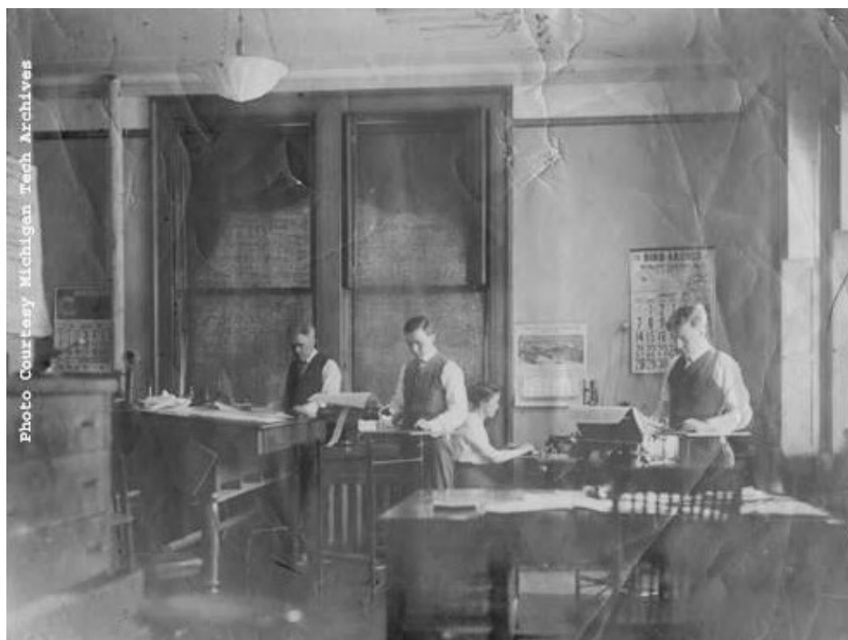
Figure 5.18: Image of men and women working on second floor of QMC office. Note the Burroughs adding machine, drafting desk, and stamp punch in the photograph. This photograph would be used to help recreate an authentic experience in the room while also providing valuable insight into the way Quincy operated. Image courtesy of MTUA/CCHC, image #: MS001.350.010.03.
