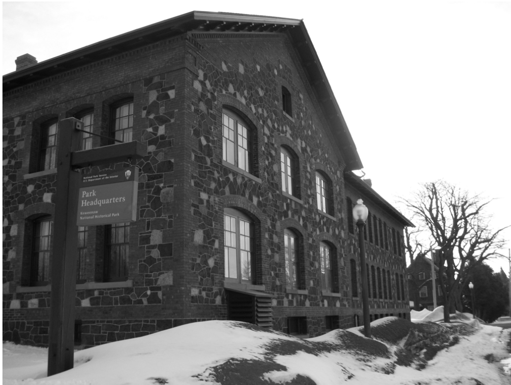
Figure 3.15: Close-up of KNHP headquarters. This is the original south side, along with the 1909 east addition in the rear. Photograph by author, 2011.
