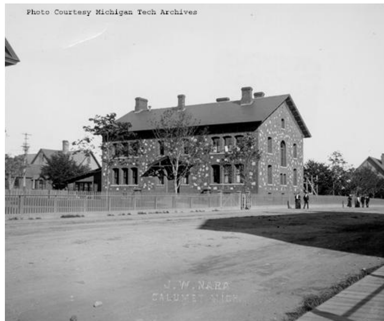
Figure 3.3: C&H general office with fence plus what appears to be scaffolding on the east side for either 1899 or 1909 addition. Image courtesy of MTUA/CCHC, image #:Nara 42-228.
