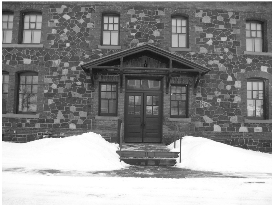
Figure 3.11: Front entrance to KNHP headquarters on the east side of the building. Photograph by author, 2011.
