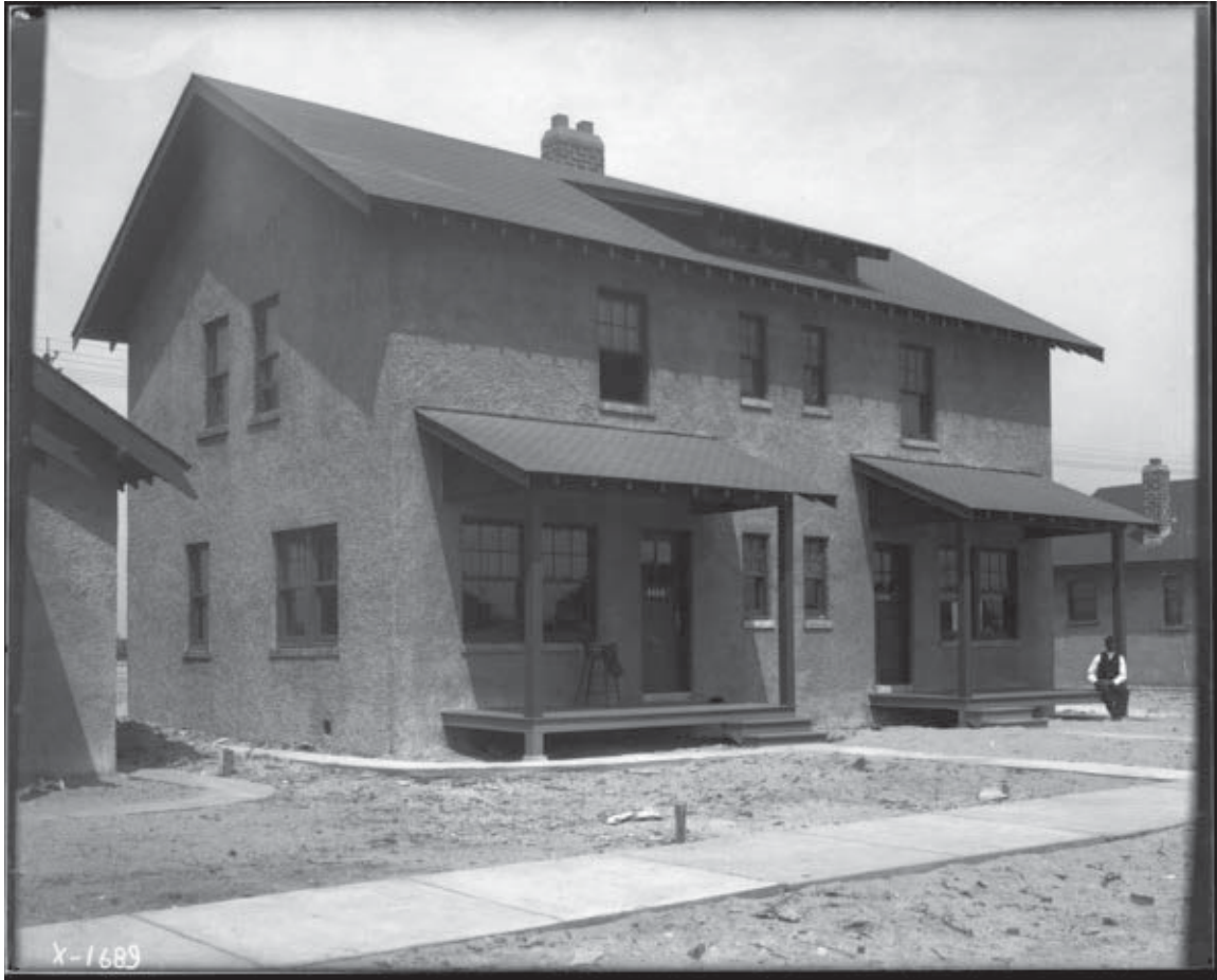
Figure 2.9 1320-24 Carolina Street shortly after construction, 1918. Courtesy of Calumet Regional Archives, Indiana University Northwest.
